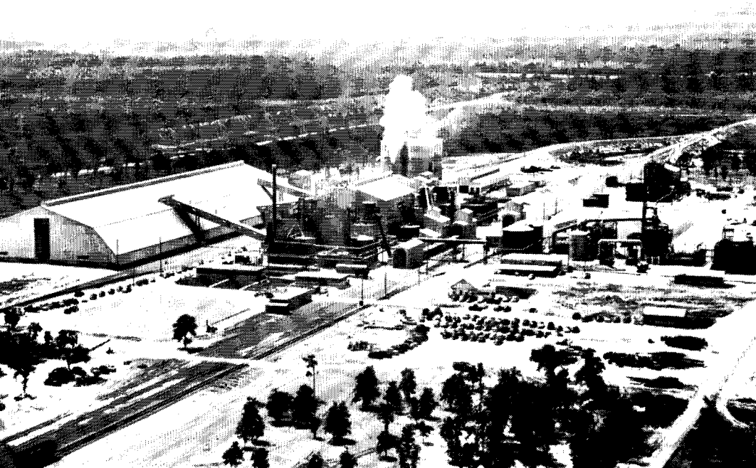
$15 million Bonnie plant at Bartow, Fla., producing animal feed supplement and plant food products. First plant in Florida for full scale recovery of uranium from phosphate rock
